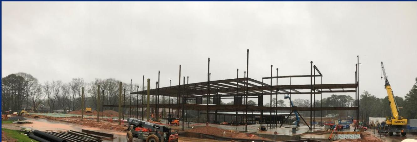
Photo of the project site with sequence 2 & 3 steel in progress
